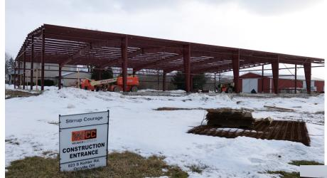
But finally at the end of January, we got word that the roof and siding were coming in, and the steel framing was ready to go up for our building! You can really get a feel for the size of the facility with the frame up next to the existing red storage barn!
